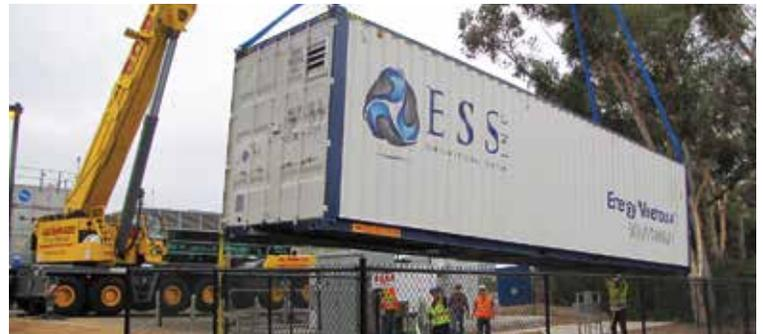
An Energy Warehouse is operating as part of an advanced microgrid at University of San Diego, CA. With its small footprint and non-toxic, non-flammable chemistry, the system was easily sited on the campus.
